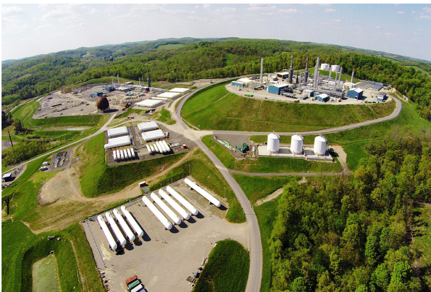
Markwest’s Houston complex in the Marcellus has the ability to process 355 MMcf/d of natural gas and fractionate 60,000 Bbl/d of liquids.
