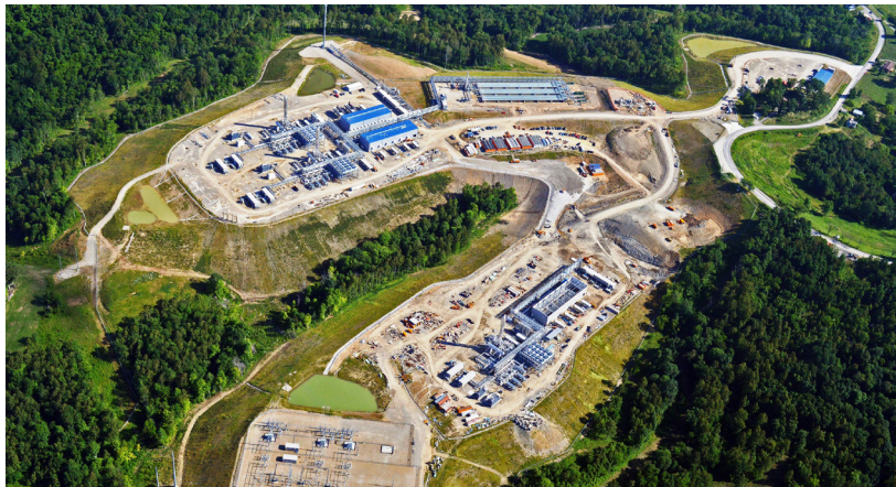
Markwest's Seneca complex can process up to 600 MMcf/d of gas from the Utica Shale.
